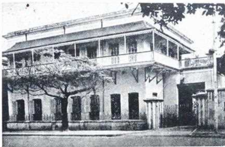
SOUTH SUBURBAN COLLEGE 26, Lansdowne Road. THE FIRST OF ITS KIND IN SOUTH CALCUTTA. The nucleus of Asutosh College 1916-1917
